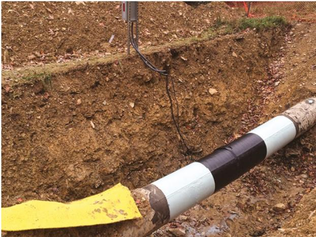
Figure 1: Fully coated and wrapped installation with RS-485 cable mounted in test station for data collection.
